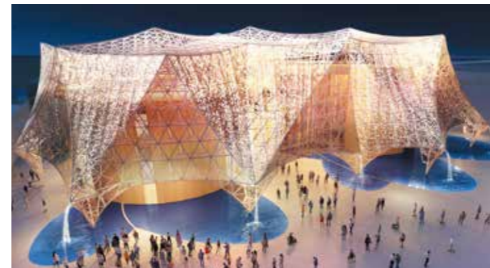
Provided by: EXPO 2025 Osaka Pavilion Association
