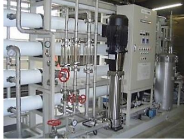
Water treatment equipment
