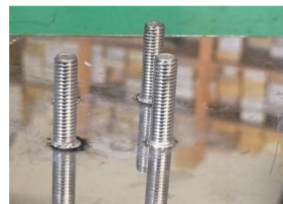
〈Step 3〉 Welding is completed.
