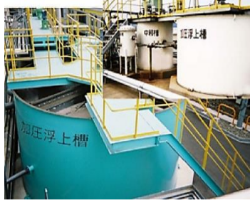
Drainage treatment equipment
