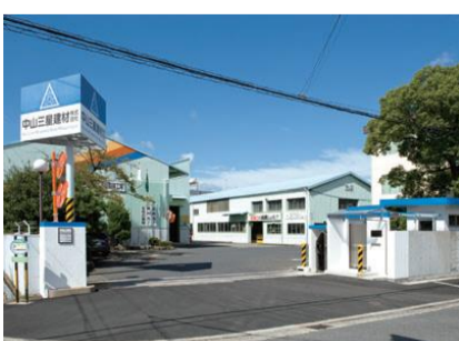
Entrance of Head Office
