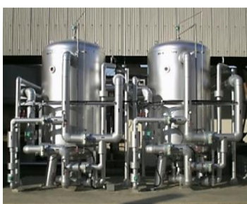
Iron/manganese removal equipment
