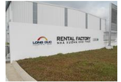
Vietnam Factory in Long Duc I.P., Dong Nai Province
