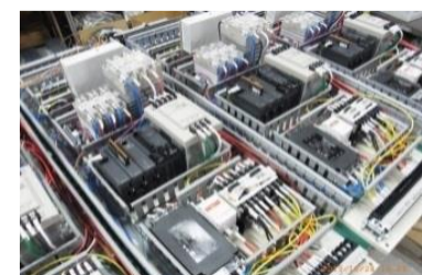
Assembly of power-supply box
