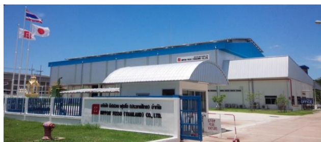
Nippon Fusso Thailand Head Office / Factory Eastern Seaboard Industrial Estate (Rayong)
